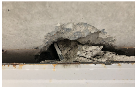
Fig. 10. Destructive shape of shear connector
