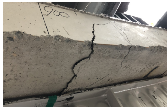
Fig. 11. Destructive shape of concrete slab
