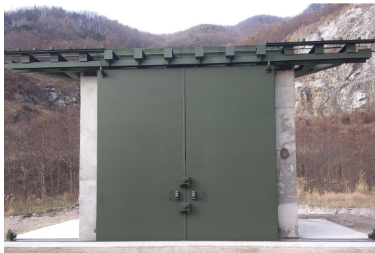
(b) Sliding door installed outside
