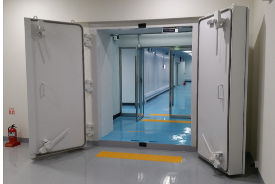
(a) Swing door installed inside
