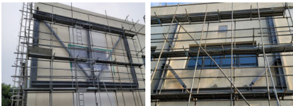
Fig. 5. Buckling restrained braces configuration
