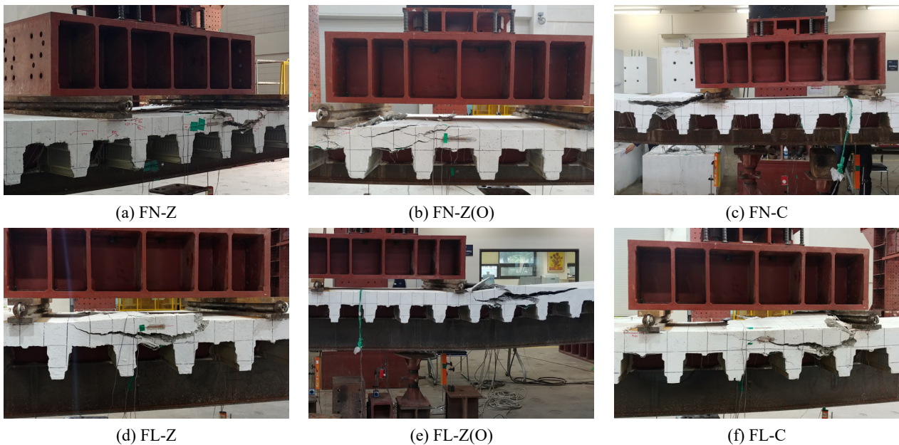
Fig. 6. Failure modes of beam specimens
