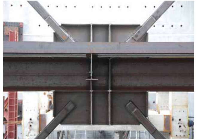
Fig. 3 Mid-span gusset plate connection detail
