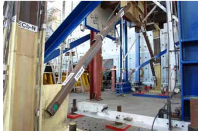
Fig. 11 Fracture of 1 st floor braces
