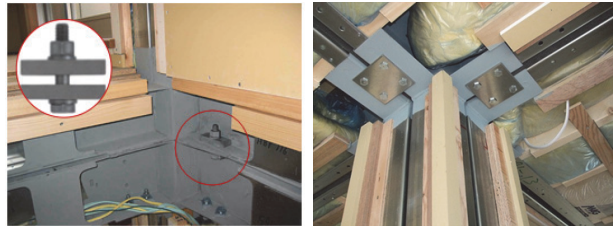
Fig. 2. Connection system of Sekisui Heim
