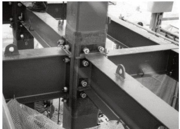
Fig. 1. Connection using TBB (twist off blind bolt)<sup>[4]</sup>
