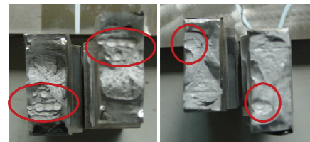
Fig. 1. Weld defects of high strength steel joint [1]
