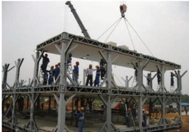
Fig. 1. Dongting Lake Hotel with 2D structural system using floor cassette to column connection example (Liu, Xuechun et al, 2017)
