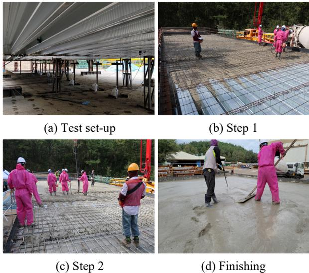
Fig. 7. Test procedure for concrete casting test
