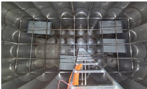
(b) Example of additional horizontal reinforcement frame
