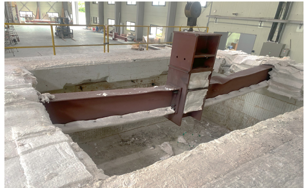
(b) Insulation of tension flanges and column interior
