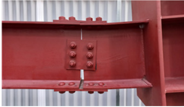
(a) Joint after the test
